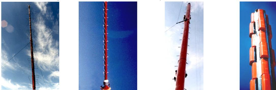
Fig 11 – High gain antennas used by TV transmitters
